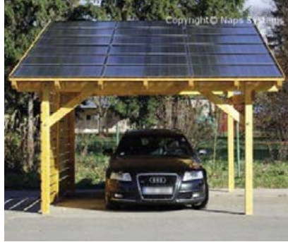
Carport solar structure
