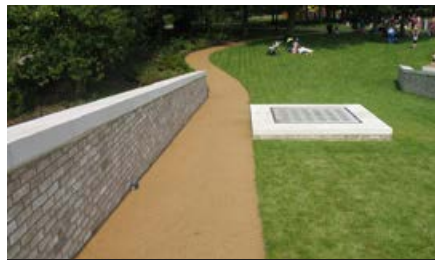
Resin bound surface for narrow pedestrian links.
